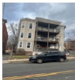
Exterior View of the Subject
